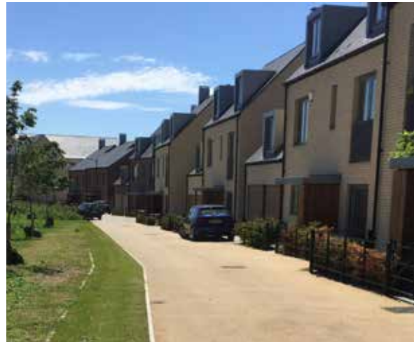
Shared surface lane providing access to properties
