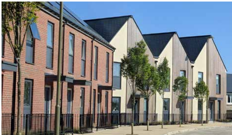
Terrace properties at Elmbrook, Bicester
