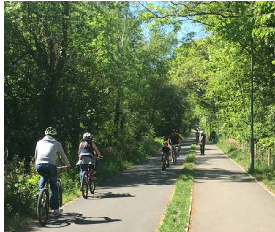
Lit off-street route containing footway and cycleway
